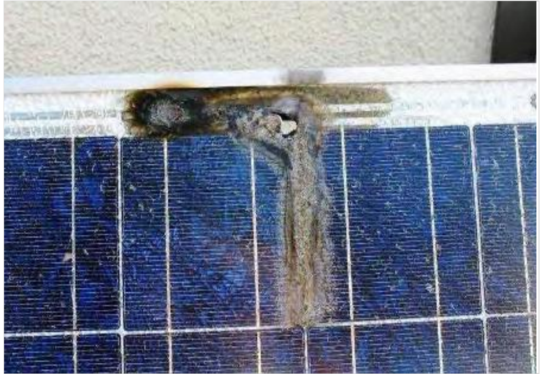
Figure 3.5 Module Failure Mode: Hot Spot
