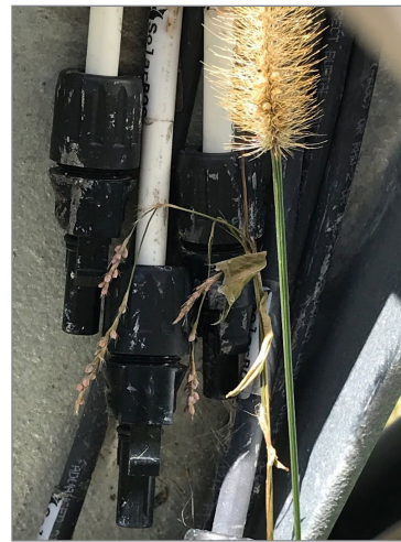
The connectors above are examples of potential time bombs: they were left unplugged without end caps at a utility-scale plant (left) and a commercial rooftop system (right).
